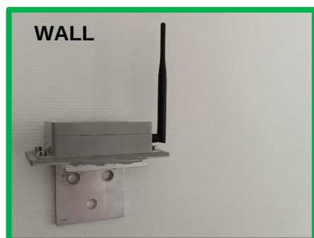
Fig.5 : good installation (front view)
